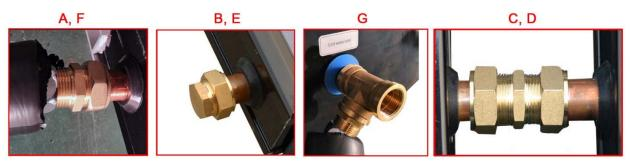
If solar water heater is equipped with two or three units of solar collectors, please see the connection of two solar collectors from the marks C and D.
